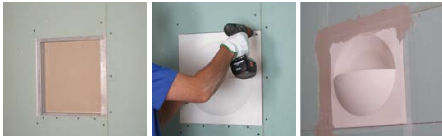
Druga metoda montowania / The second method of mounting
